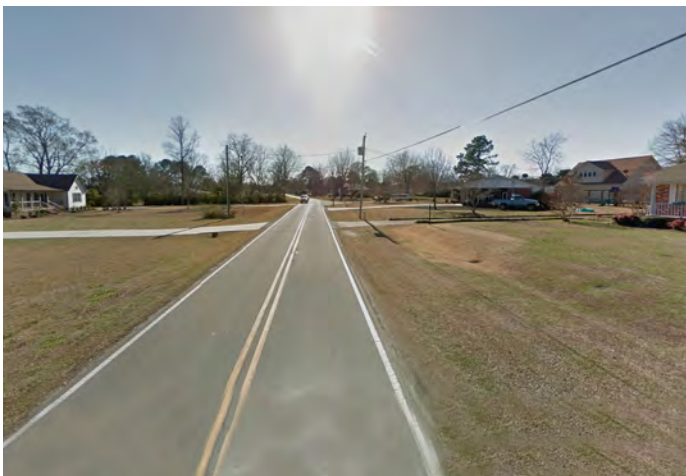
Existing conditions on Church Street (looking south) where sidewalks are lacking on both sides
