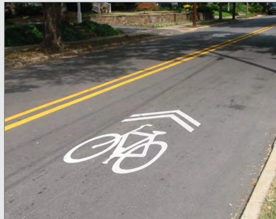
Example of shared-lane markings on pavement.
