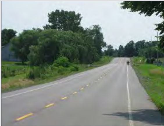
Example of 5' wide paved shoulders.
