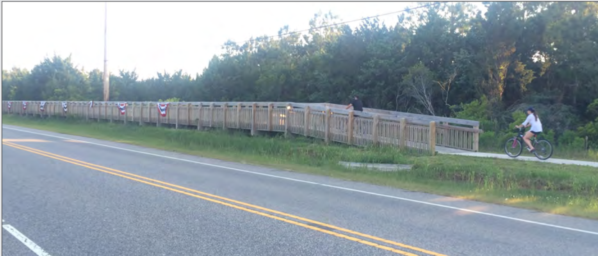
Sidepath example using boardwalk along a roadway in the Outer Banks, NC.
