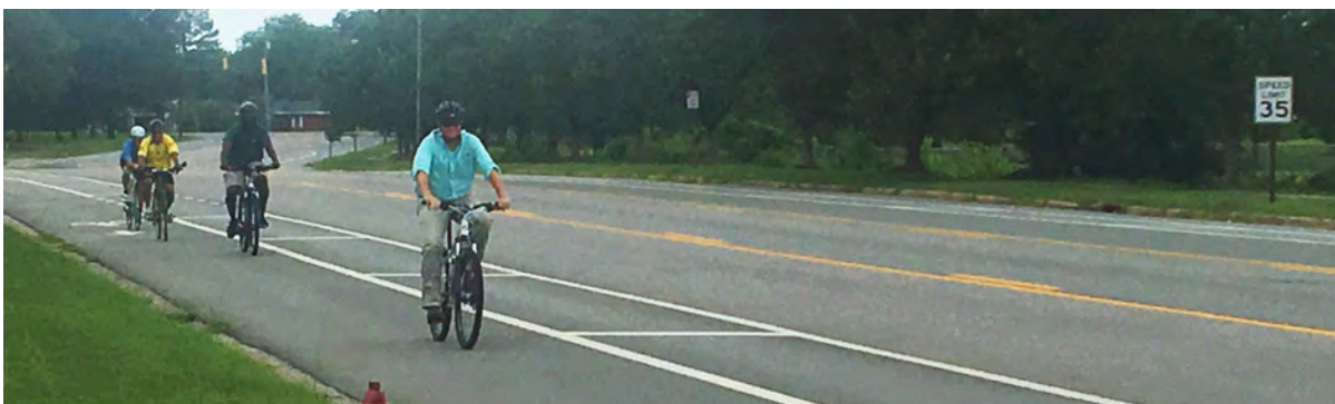
Coordination with a recent repaving project in Goldsboro, NC, allowed for an opportunity to restripe the road with buffered bicycle lanes, as shown above. This was a recommendation that came out of Goldsboro's Bicycle, Pedestrian, and Greenway Plan.
