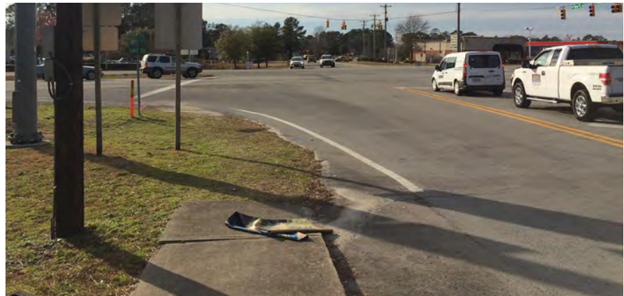
The sidewalk on Howard Boulevard ends before reaching the intersection at US 70. Crossing improvements to get across US 70 are lacking.
