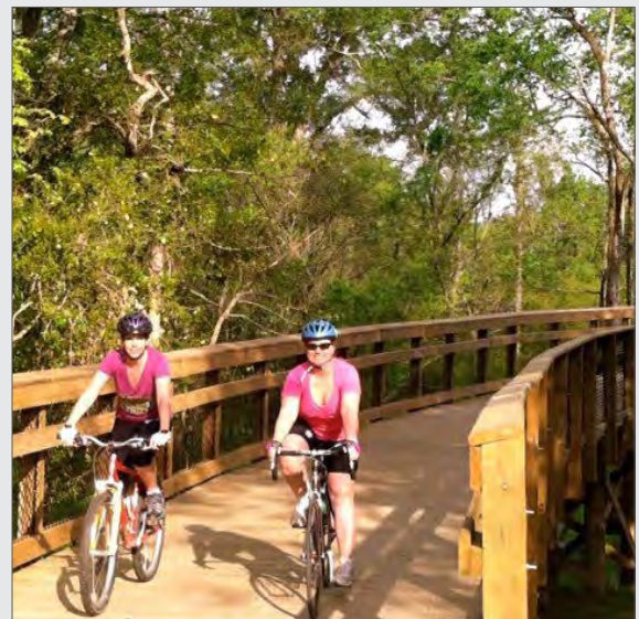
Boardwalk can also be used for shared use paths in wetland areas, or areas prone to flooding.
